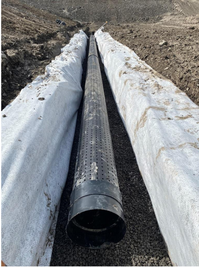
Photo 12 Under-cell Drainage Pipework at Existing WMF, June 2022
