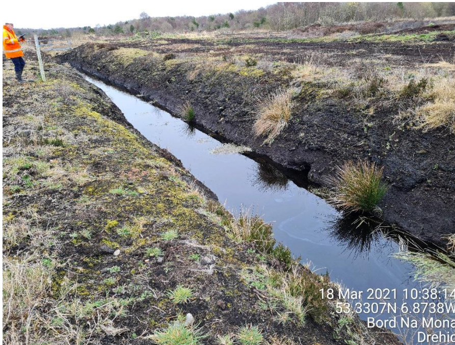
Photo 2 Exposed Peat Along Drain Near the Landfill Expansion Area
