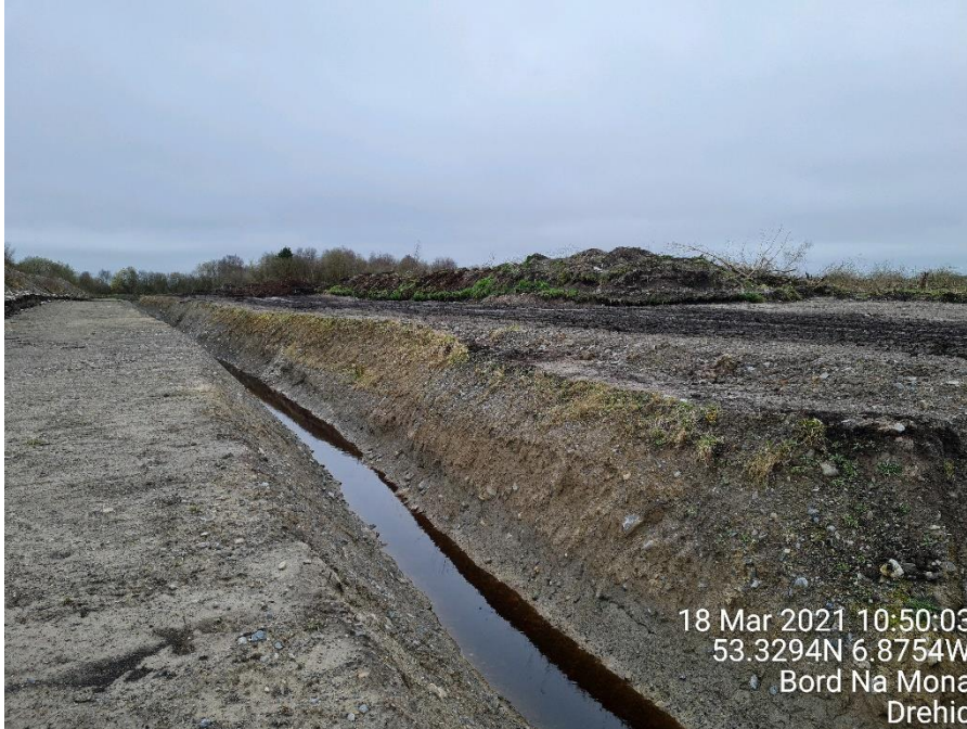
Photo 9 Drain Extending into Subsoils and With Adjacent Peat Stripped
