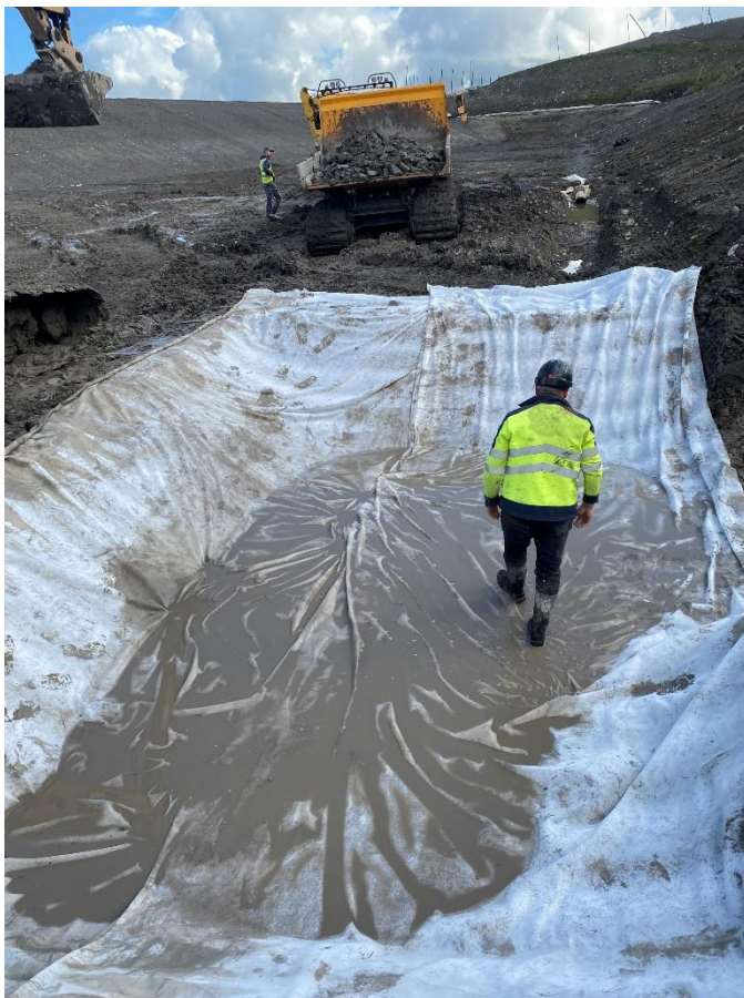
Photo 11 Sump Inside Excavation at Existing WMF, June 2022
