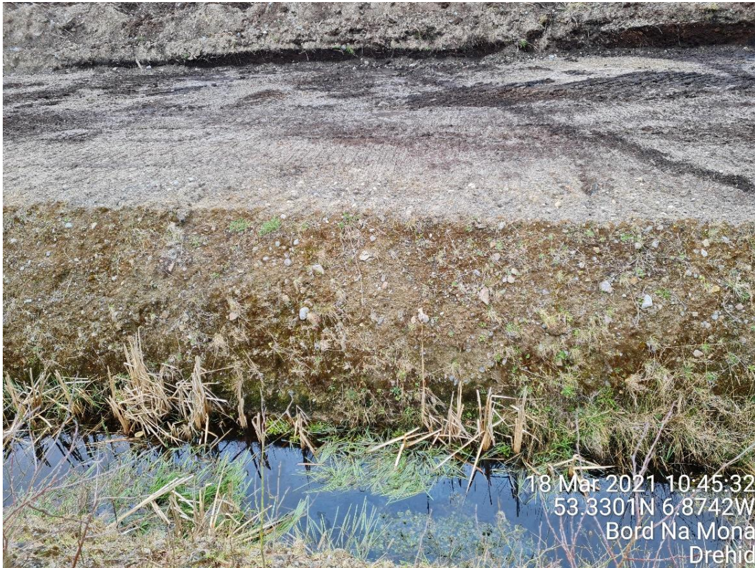
Photo 3 Exposed Subsoils Beneath Stripped Peat Near the Landfill Expansion Area
