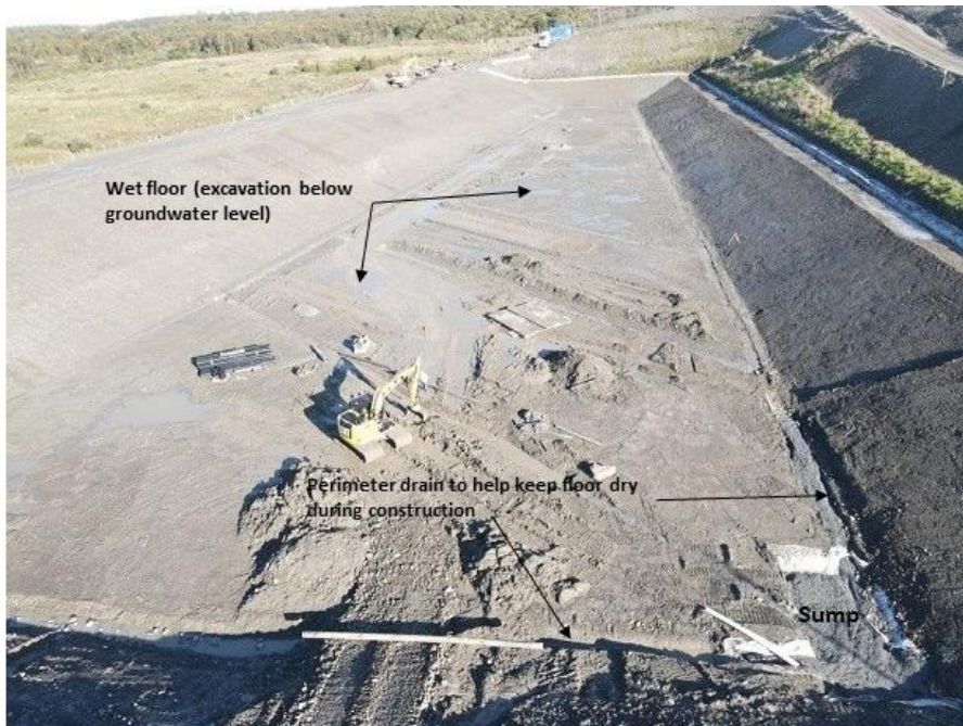
Photo 10 Perimeter Drain Inside Excavation at Existing WMF, June 2022
